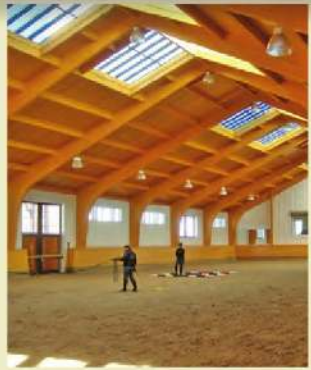
Venting cupolas, clerestory windows, skylights, and sliding barn doors in a riding ring make for a pleasurable indoor riding experience in Long Island, New York.
